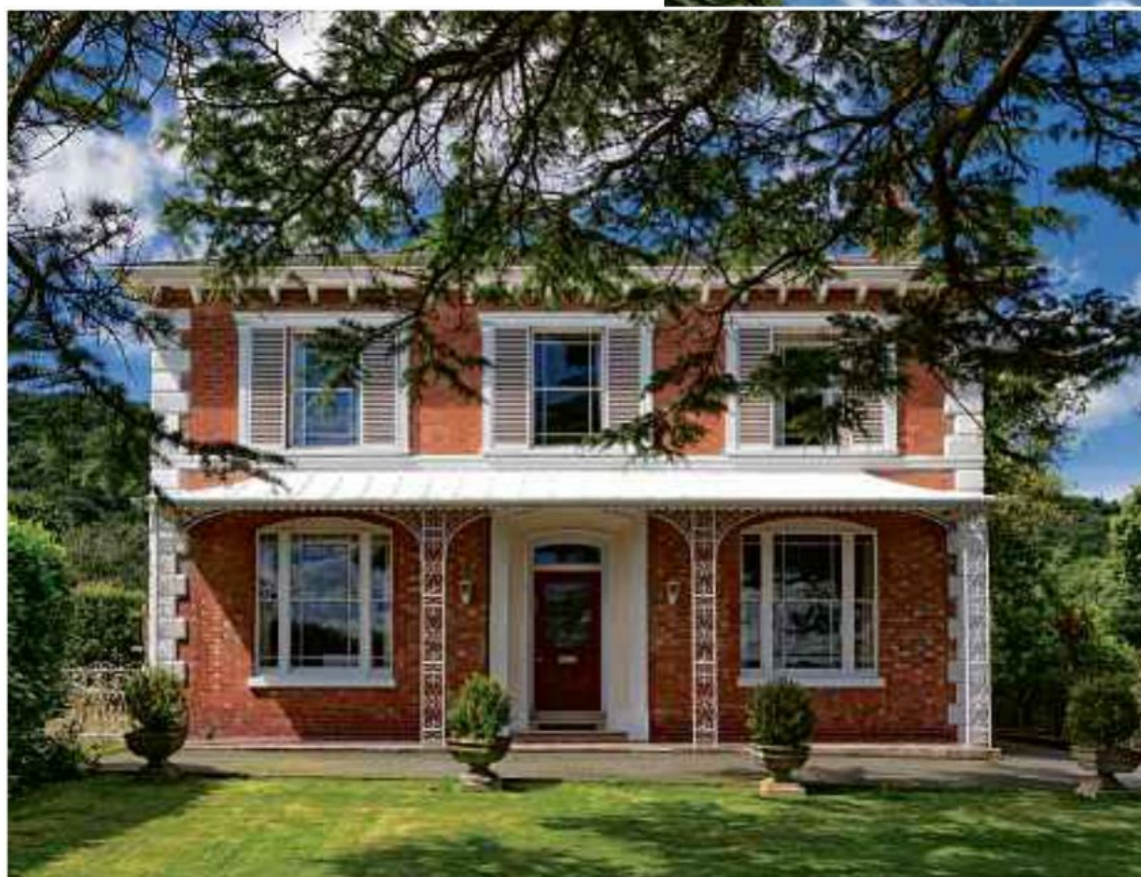
▶ South Bank, Middletown, Welshpool, Powys. A detached village house in an elevated position with views towards Long Mountain. It was extended in 1872 to include the cast-iron veranda at the front. It has high ceilings and period fireplaces, and the mature gardens include a wildlife pond and a fruit orchard. 4 beds, 3 baths, 3 receps, conservatory, outbuildings, 1 acre. £595,000 Savills 01952-239500.
